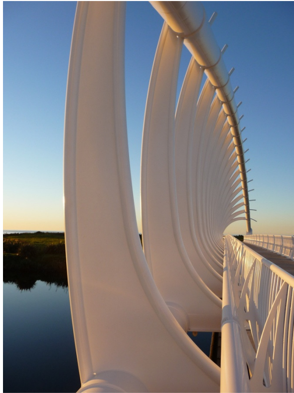
Figure 6: An aspect of the Te Rewa Rewa Bridge showing the tubular arch forming a gateway. The coast horizon of the Tasman Sea is in the background.
