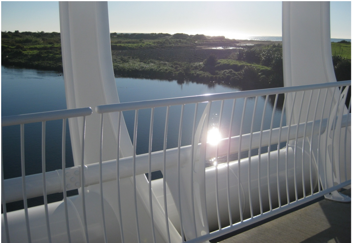
Figure 5: The coastal horizon and the natural flood channel of the Waiwhakaiho River showing the proximity of the bridge to the Tasman Sea.
