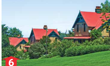
▲ Here are the original Worker's Cottages as they stand today.
