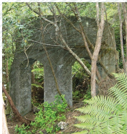
Remains of the concrete foundations that supported cyanide vats, Golden Hills Battery.
