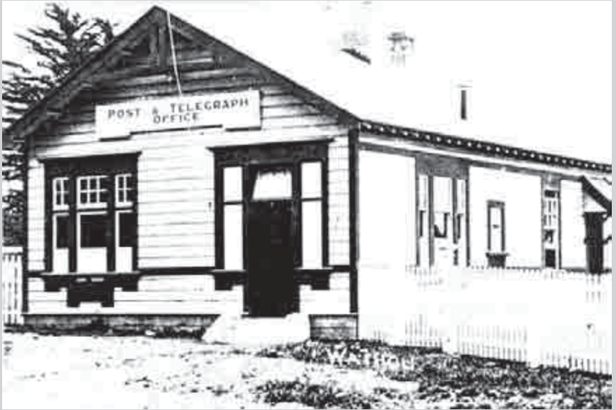
Site 56: Waihou Post Office.
