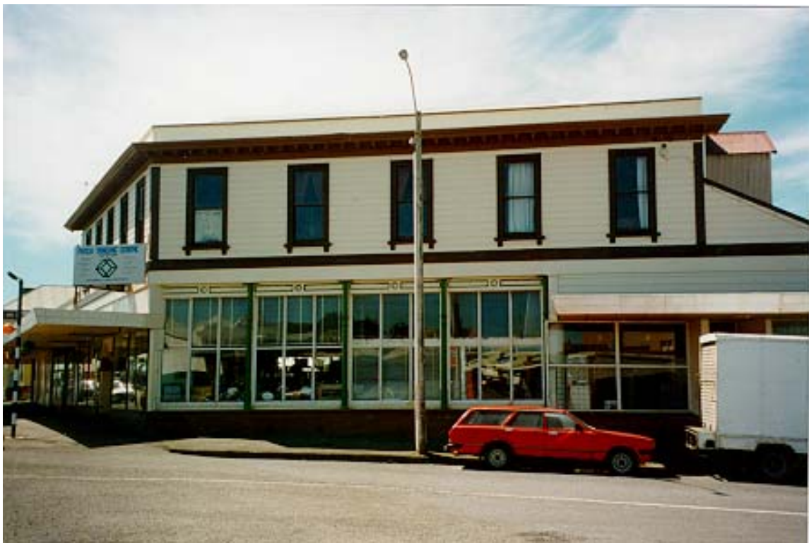
Leicester Street façade of the former Gibson Store building
